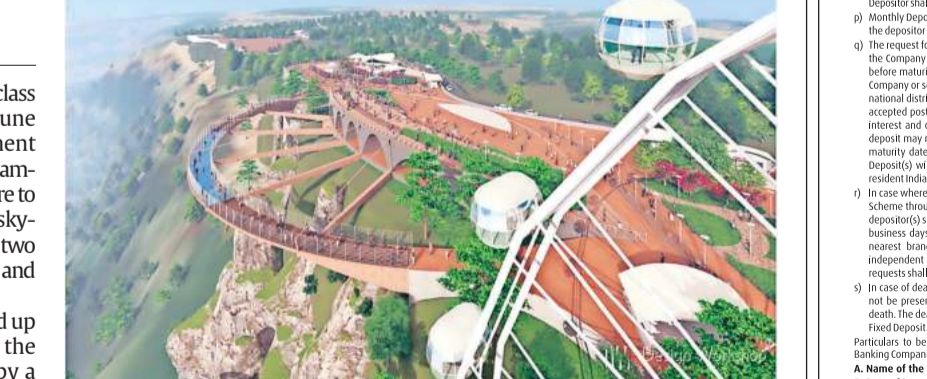
The project includes construction of a six-metre-wide and 90-metre-long bridge, but the main attraction would be the 125-metre long and six-metre wide skywalk. Express
