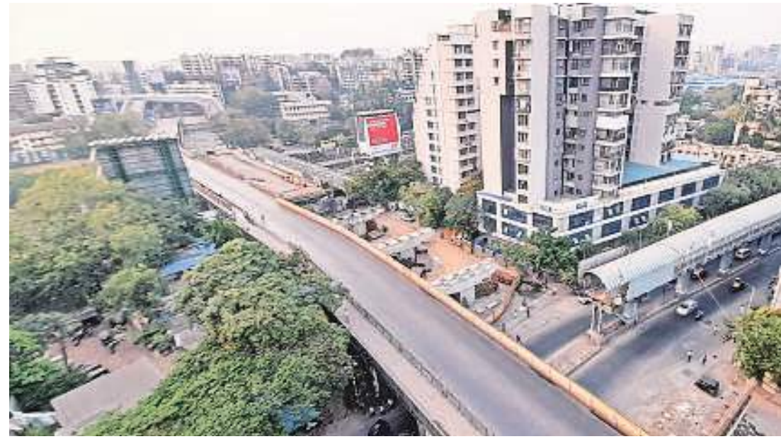
An empty Gokhale Bridge after it was closed on Monday. Pradip Das
